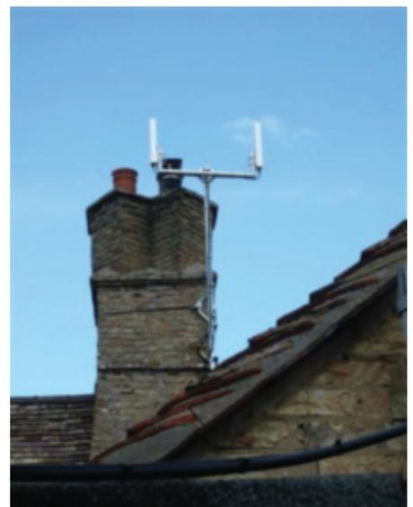
Figures 03 & 04: TVWS antennas, installed at the ADC theatre and at one of the pubs
